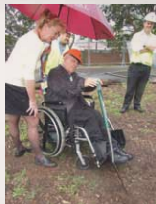
Ron Cowland turns the first soil.
